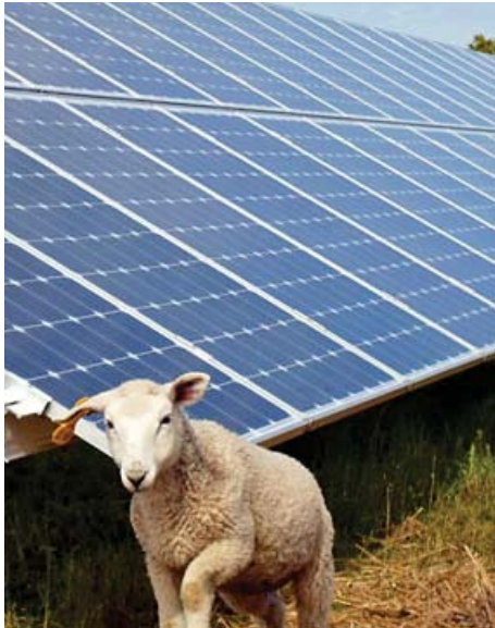
At PCC Rock Creek sheep graze along side PV array powering the campus
