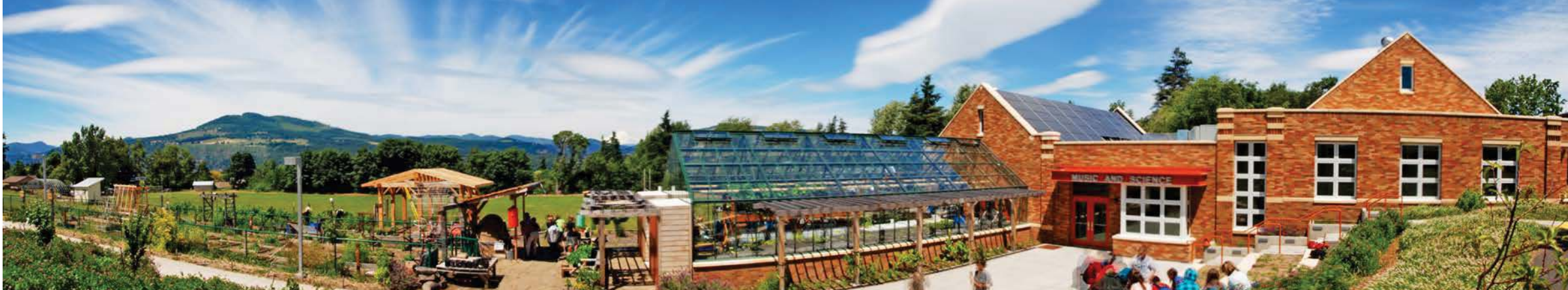
Hood River Middle School learning garden, green house and rooftop PV array
