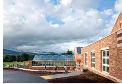
First public school to earn LBC Net-Zero Energy Bldg Certification National AIA COTE Top 10 Award LEED Schools Platinum Certification 35 kW PV array producing 35,000 kW/yr
