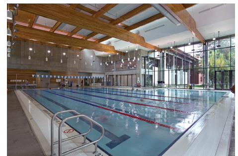
Extensive daylighting keeps the natatorium bright and welcoming. In this construction view, the pool is well-lit prior lighting fixture installation.
