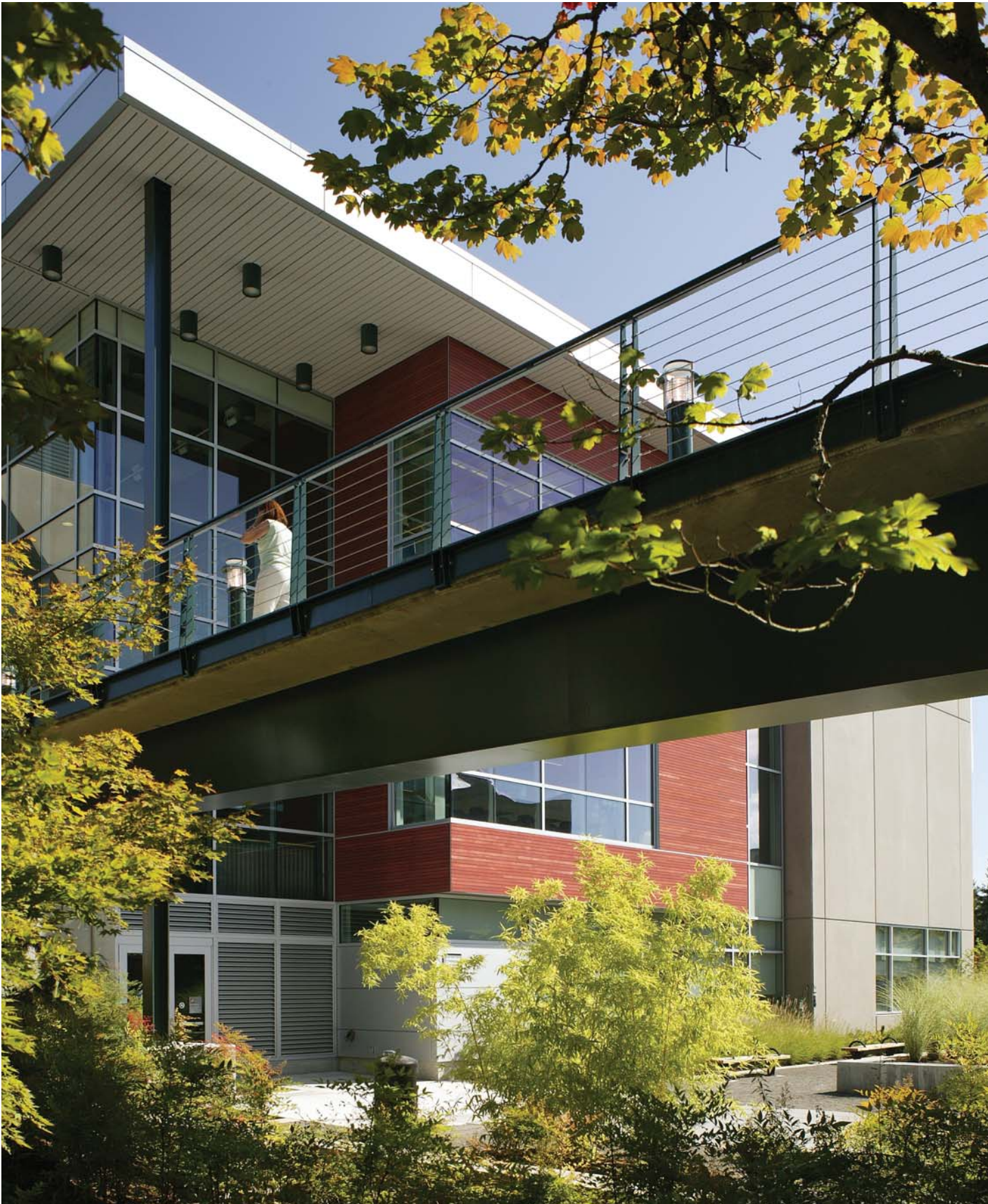
technology classroom building portland community college portland, oregon
