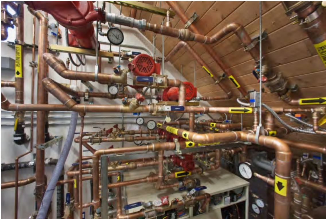
Mechanical system pumps and pipes fill the mezzanine space and can be seen through a window from the science classroom below.
